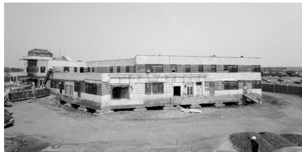
Historic building 51 being moved to new airport location to allow runway expansion
